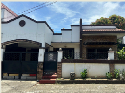
Original Property Condition
